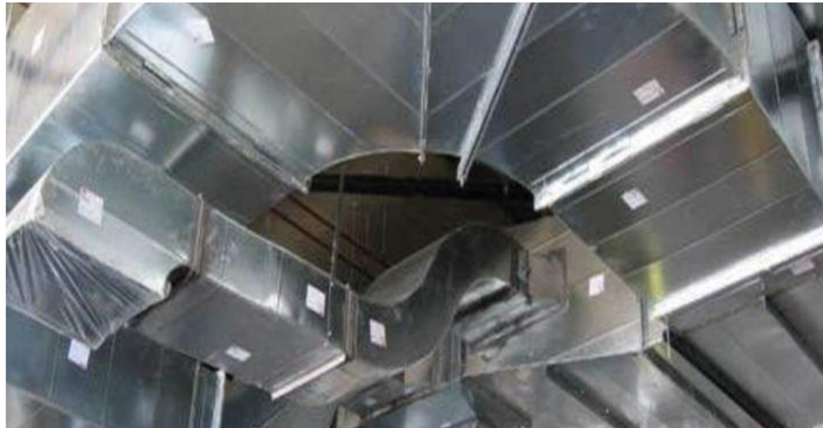
M S AND S S DUCTING INSTALLATION
